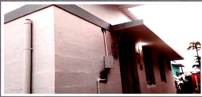
As a mark of the Diamond Jubilee Celebration, a new house was constructed for Mr.M.Mani, Watchman and the house warming ceremony was held on 14.04.2022.
